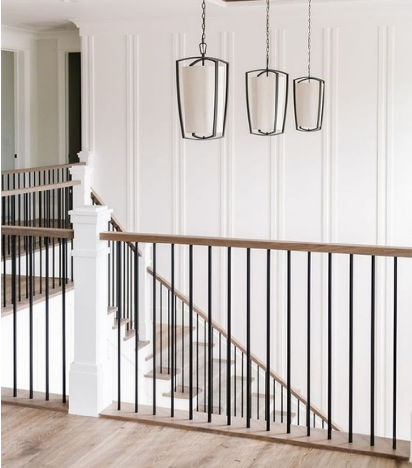
APPLIED FLAT TRIM ON ALL WALLS
