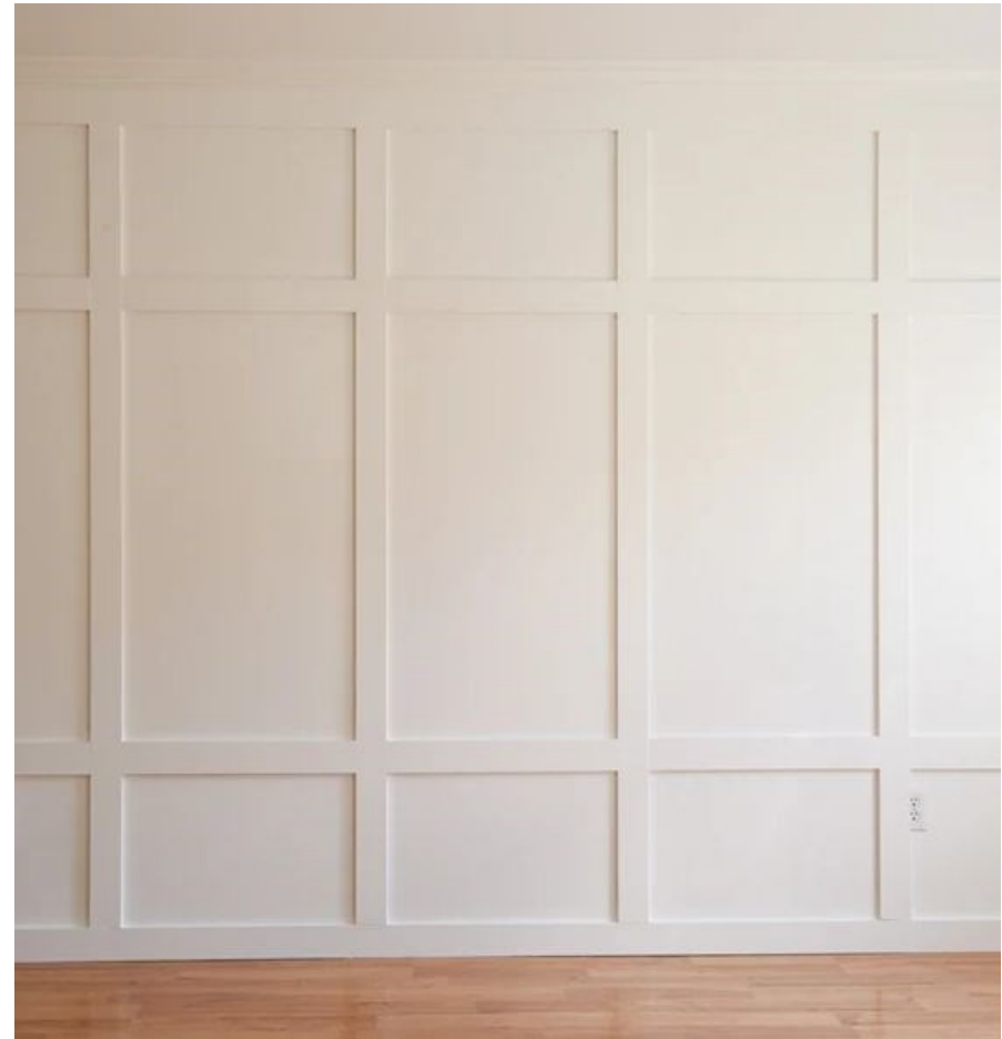
APPLIED WALL TRIM
